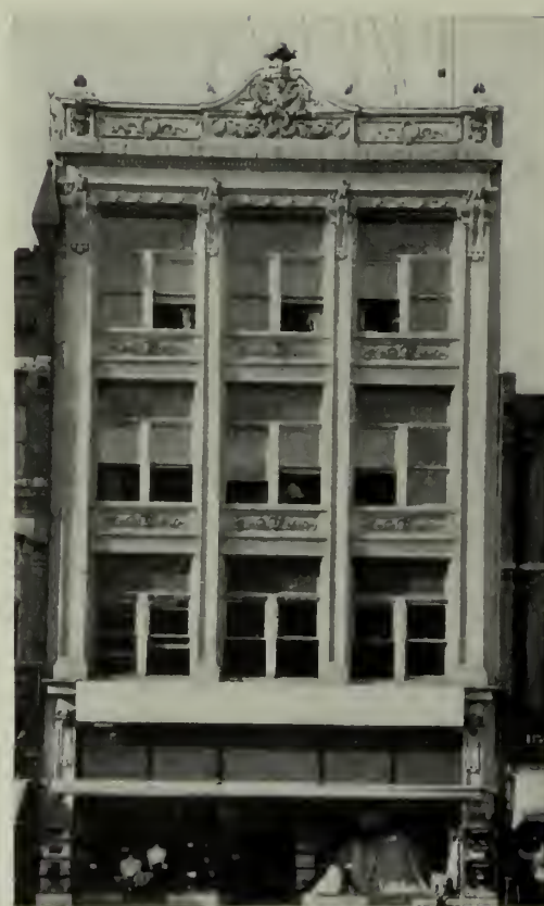
STORE BUILDING, INDIANAPOLIS. All terra cotta front executed by Indianapolis Terra Cotta Company. D. A. Bohlen & Son, Architects.
